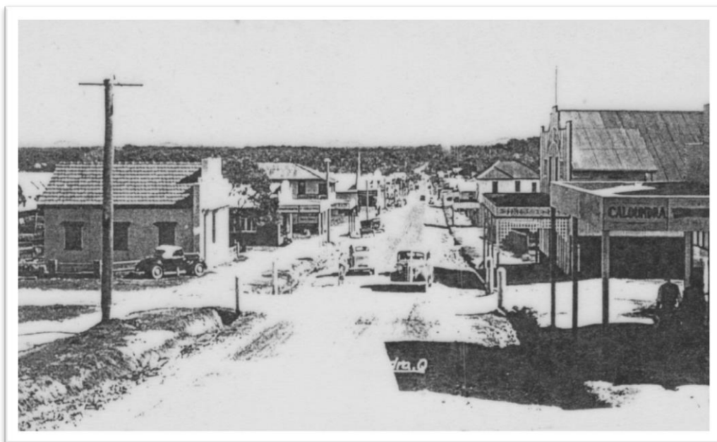
Photo 11. Bulcock Street, Caloundra, mid 1930s. The facade of the Strand Theatre, right, was subsequently upgraded in 1936. Bulcock Street is not curbed and channelled.
