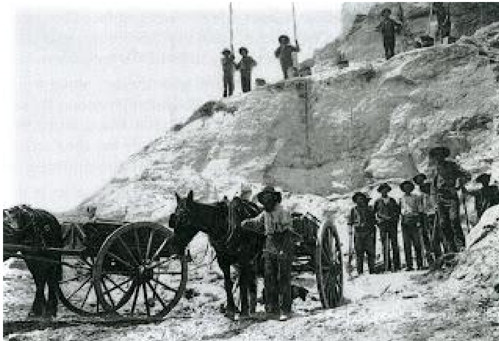
Road building across Blue Mountains, 1860s
